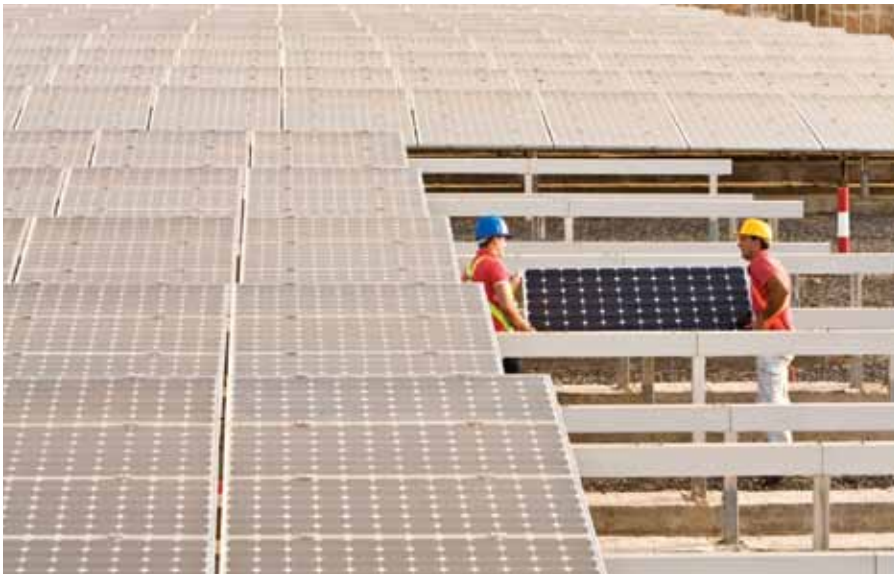
SunZia will create job opportunities through construction of two transmission lines, and through SunZia's ability to foster development of local renewable energy projects.
